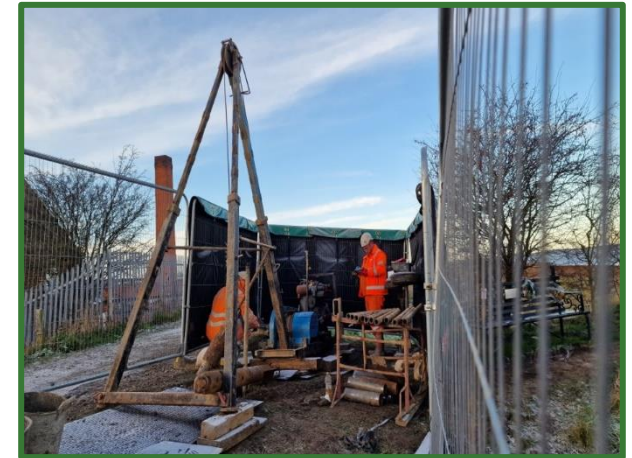
Figure 1: The project team on site using a cut down rig.
