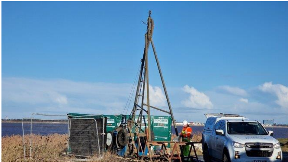
Cable Percussive Borehole – Full Sized Rig
