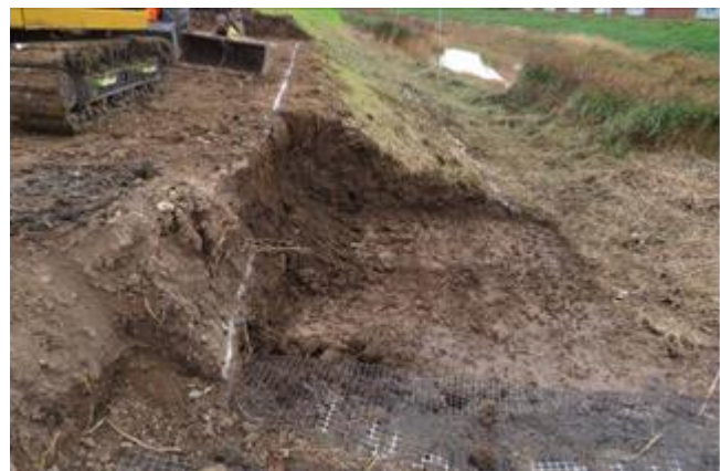
Figure 2: Grout injection repairs being undertaken near the Old Mill.
