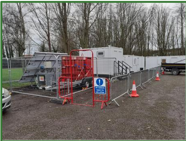
Figure 2: One of the Hydrogen Cells used to power the site.
