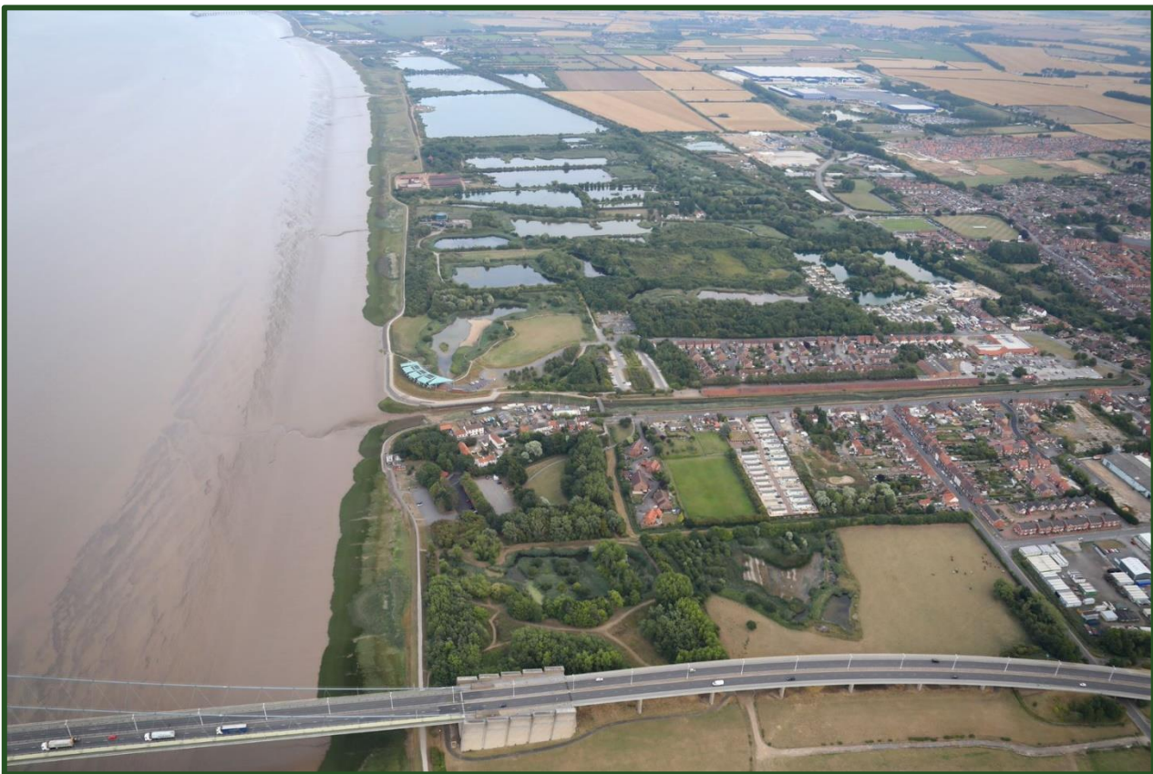
Figure 3: Drone image taken of Barton frontage above the Humber Bridge looking eastward towards New Holland.
