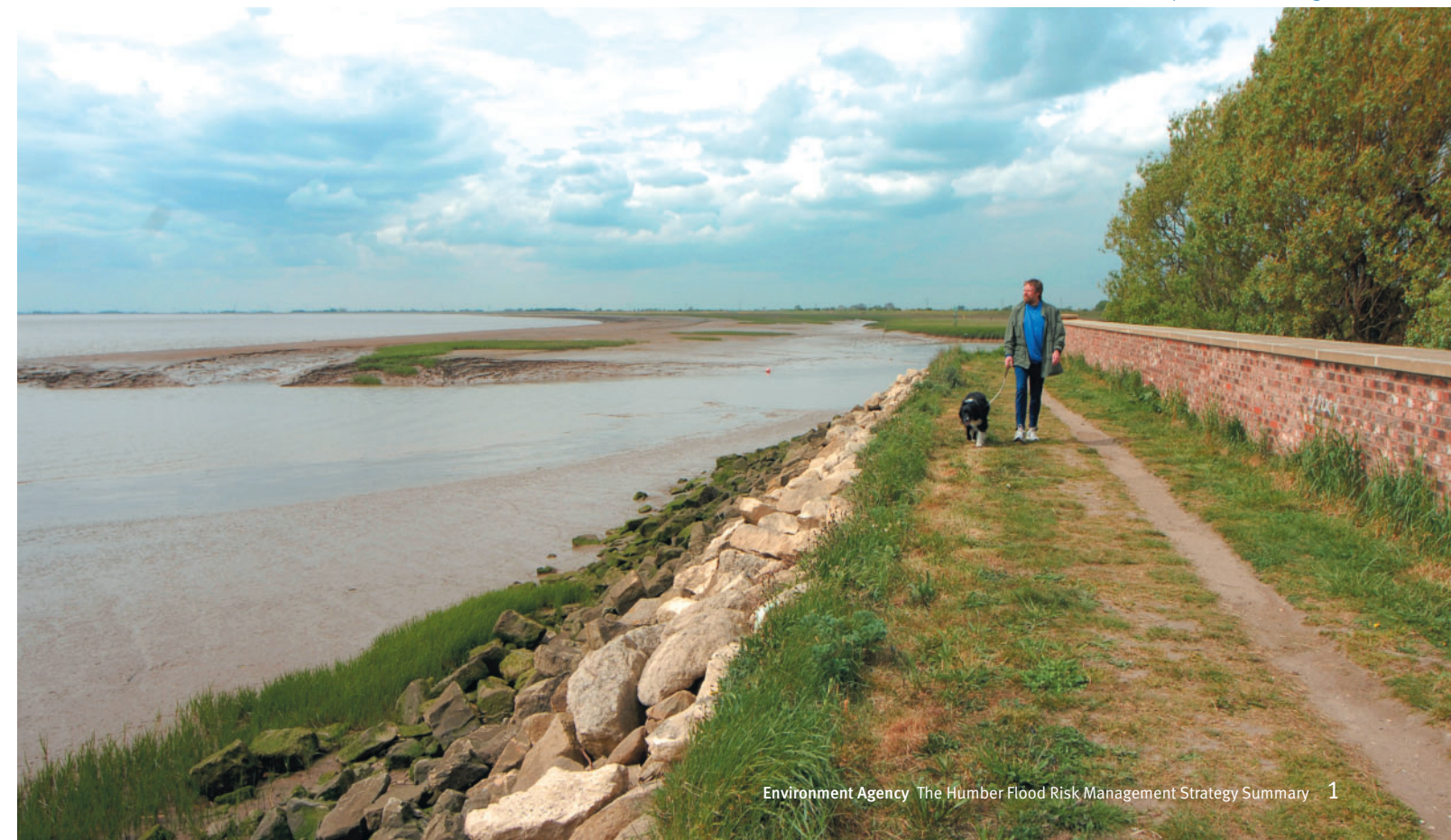
Flood defence at Brough
